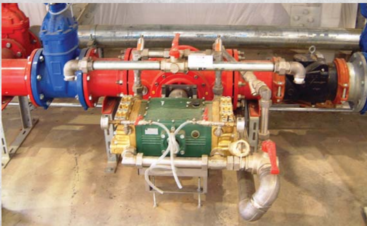
Water-Driven Proportioner Concentrate Control System
