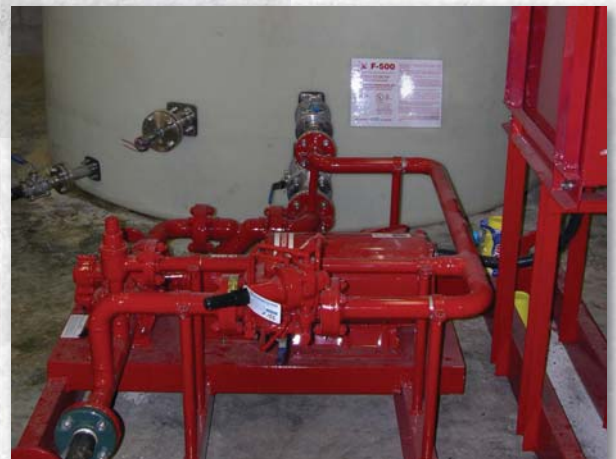
Balanced Pressure Pump Concentrate Control System
